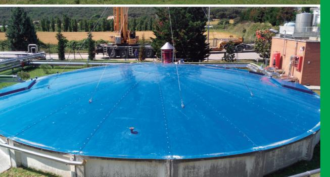
Our covers are characterized by having a high mechanical resistance with a low specific weight, being fast to assemble and need a minimum maintenance.
